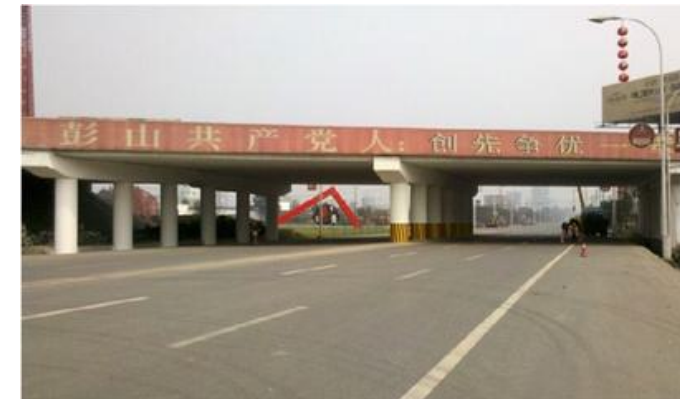
After: With Airlite Sunlight, the overpass remained clean for 10+ years due to its self-cleaning properties while absorbing 20+ kg of NOx per year, reducing pollution and maintenance costs.
